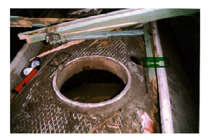
**Photograph** #4 – - Arrow shows the opening where the overflow pipe was to be welded.
