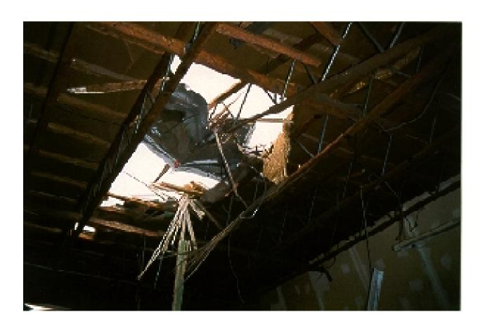
**Photograph** #2 – Shows damaged roof and cab of tank truck lodged in the ceiling.
