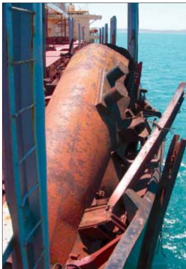
FIGURE 9: Port shoulder after the explosion
