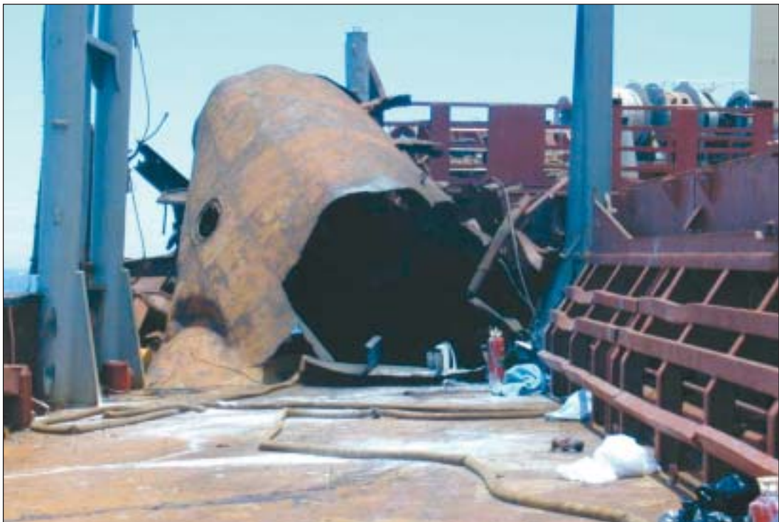
FIGURE 2: Ruptured tank on Nego Kim
