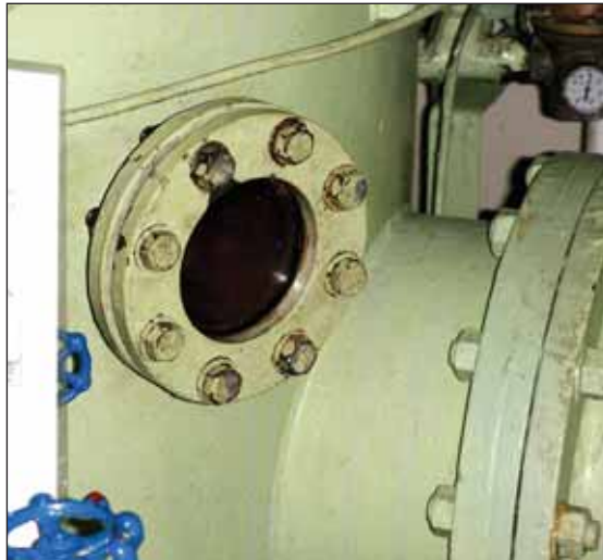
FIGURE 2: Close up of sight glass
